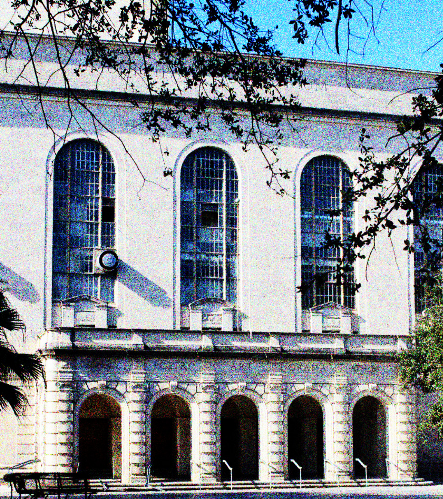
MUNICIPAL AUDITORIUM (New Orleans)
